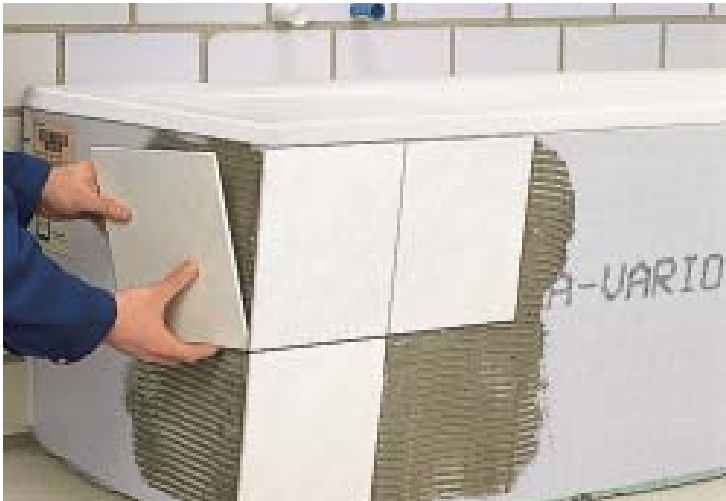
6. Tile the support. Betegel de badkuip- of douchebakdragers.
